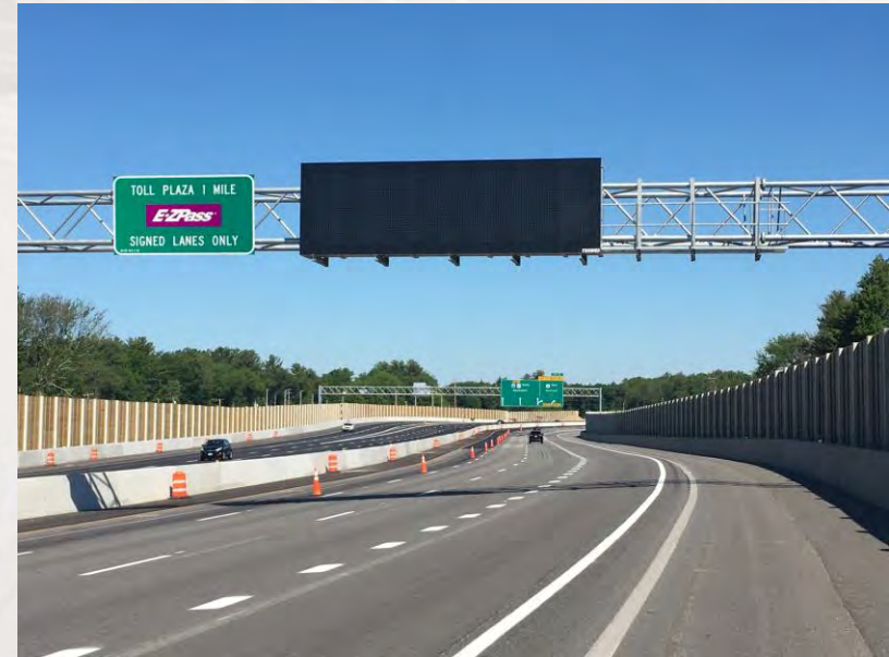
Dynamic Message Sign hanging from 190ft truss
